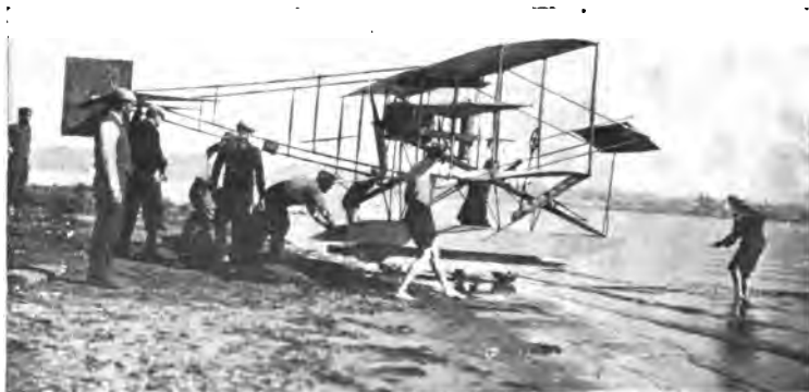
SIDE VIEW OF THE CURTISS HYDRO-AEROPLANE. SHOWING SINGLE PONTON
